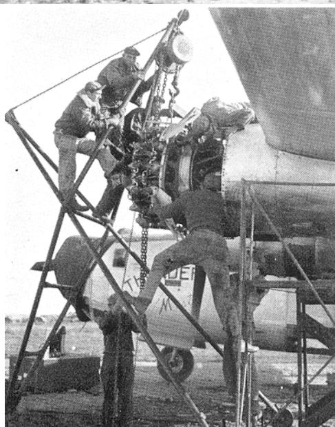
Fig. 40 The powerful engines were replaced after the required number of running hours.
